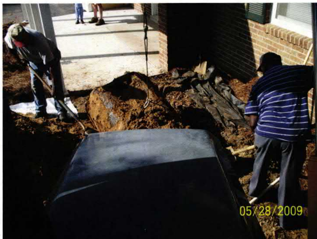
Picture 2: UST 1042Gardenia during removal.
